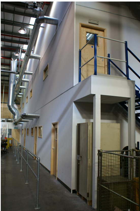
Ground & first floor mezzanine offices
