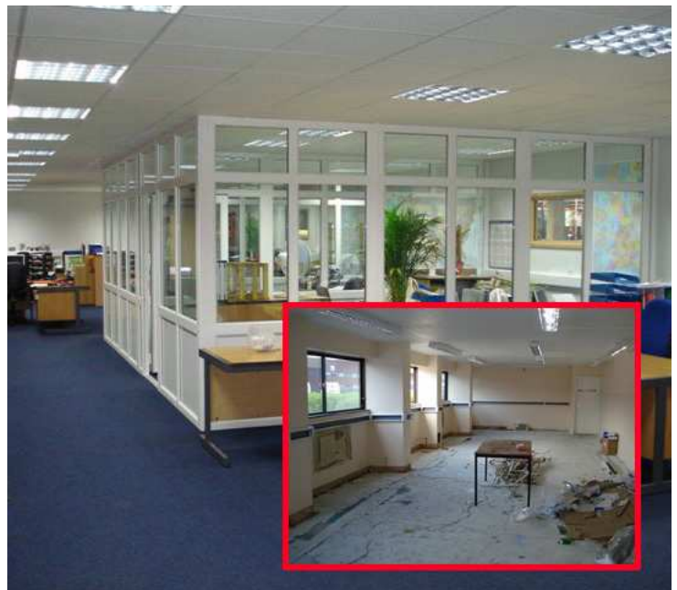
Finished offices (Main Photo), Extent of refurbishment (Inset)
